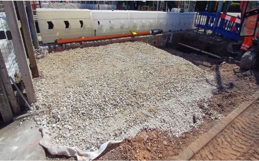
Foundation works for Platform 1 lift motor room
