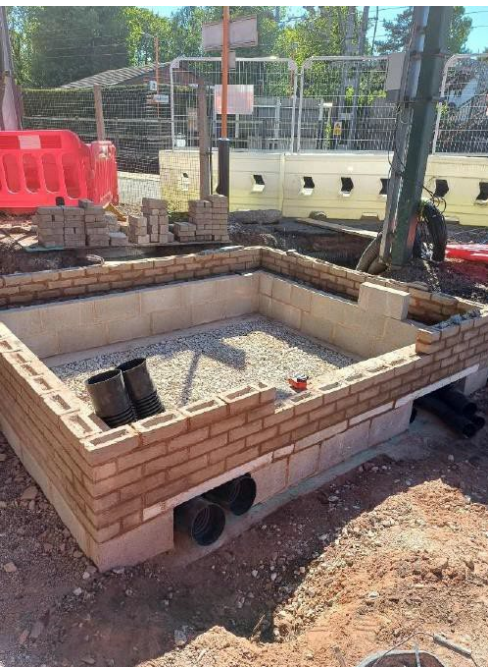
Stone for Piling mat on platform 1
